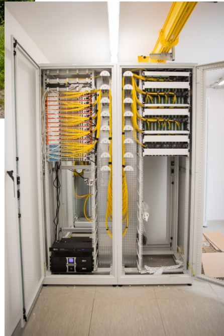
Verteilzentrale (POP, Point of Presence)
